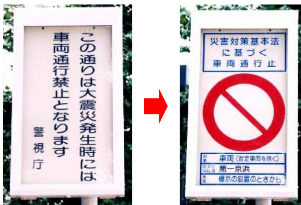
The Emergency-activated Optional Message Signpost on the sidewalks 路側式可変標識
