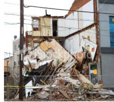
Enhanced resilience lends to reusing or even re-purposing rather than disposal due to premature collapse.
