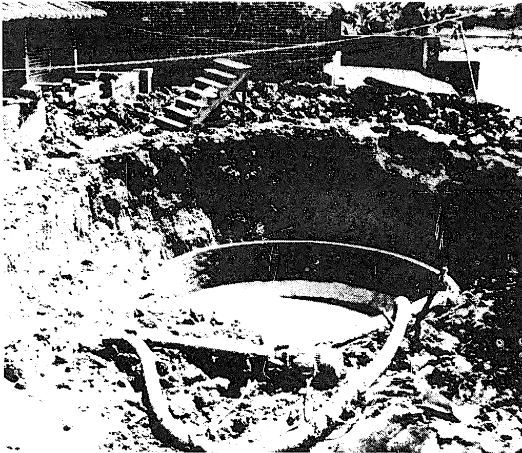
Plate II-2. 20 cu.m collective biogas pit under construction between pigsties and fishpond; 'floating construction method'.
